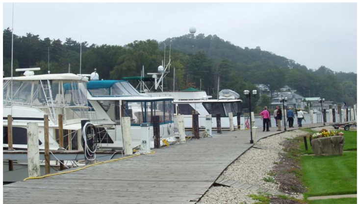
Boardwalk at Saugatuck.
