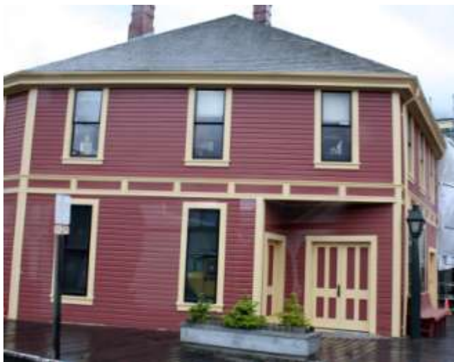
Turn of the Century building being restored.
